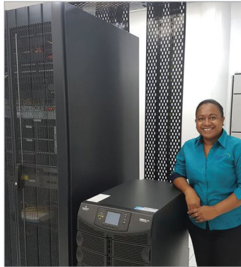
Ralema Geno, Infrastructure Manager and data centre designer, BCI
