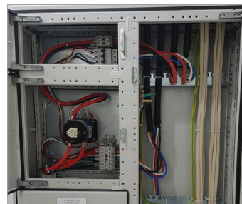
3x1 NPS customised switchboard integrated into the solution
