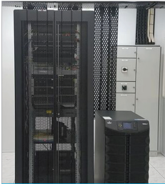
Liebert APS, rack and NPS customised switchboard
